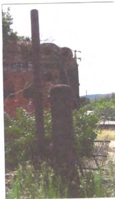
Figure 26 The blowdown tank for the boiler. The blowing down of the boiler involved opening a valve at the bottom of the boiler while under pressure allowing any mud or sediment to be discharged before it could form scale inside the boiler. The tank diffused the energy in the water by allowing steam to flash off the vent pipe and for the remaining hot water to drain away safely. (September 2010)
