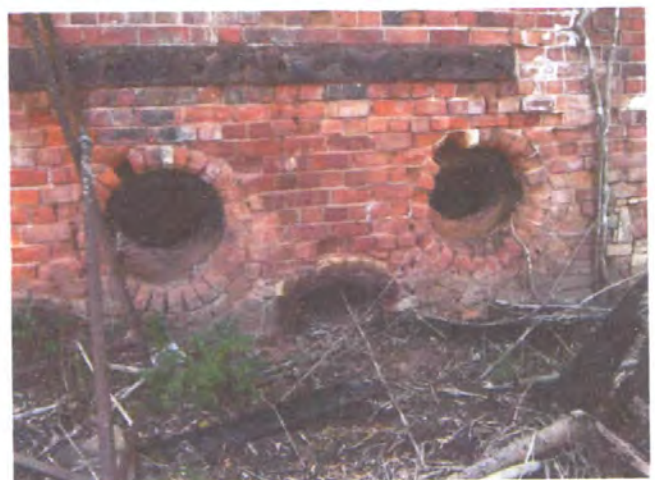
Figure 28 The water drums were suspended from above to allow for expansion, and therefore could not touch the brickwork. They were originally covered with air sealing doors (left) which are no longer present (right). These doors are visible in Figure 6. (The Stirling Boiler as used on Sugar Estates, p.12)
