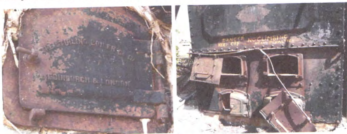
Figure 20 Left: Makers name cast into one of the access doors. Right: The original location of the centrally located oval nameplate above the furnace doors is visible (September 2010)
