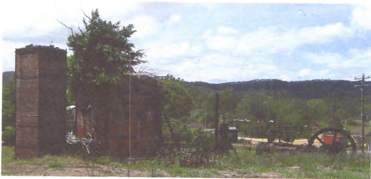
Figure 1 General view (left to right) of the chimney base, Stirling boiler, Walker's steam winch, blowdown tank, and Marshall steam engine at the Mount Molloy sawmill site (September 2010)
