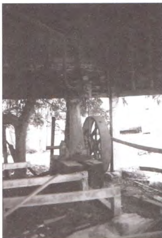
Figure 11 Tangye vertical steam engine, no longer present on site (Geoff Green, 1973)
