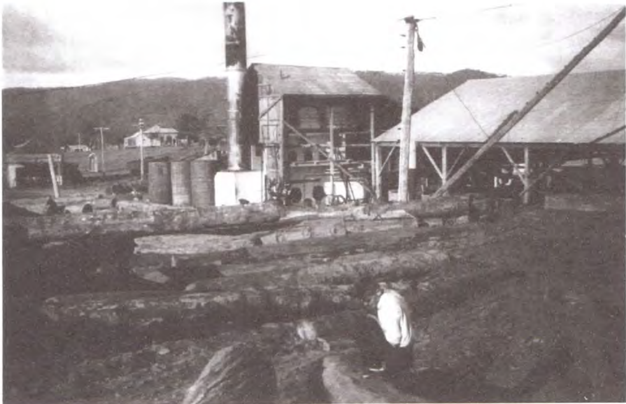
Figure 6 Mount Molloy sawmill, c.1938. The original chimney was on a shorter brick base immediately behind the Stirling boiler, and the three tanks next to the chimney held water for the boiler. The boiler was housed in an open sided building with the brickwork painted white. The flywheel of Marshall engine is visible in shed on the right the Walkers winch is visible in front of the boiler along with associated stiff leg derrick crane. Wagons on the railway line are visible to the left of the boiler house (Cairns Historical Society, P12831)
