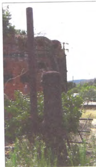
Figure 26 The blowdown tank for the boiler. The blowing down of the boiler involved opening a valve at the bottom of the boiler while under pressure allowing any mud or sediment to be discharged before it could form scale inside the boiler. The tank diffused the energy in the water by allowing steam to flash off up the vent pipe and for the remaining hot water to drain away safely. (September 2010)
