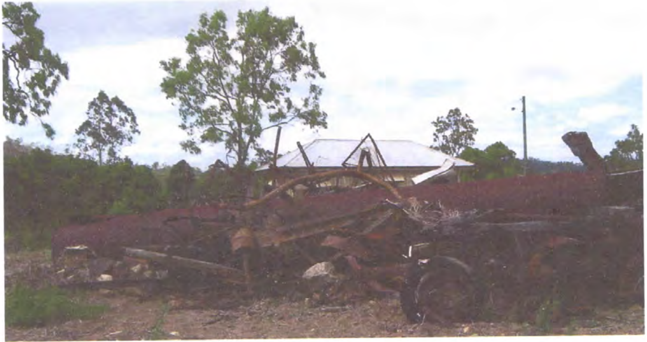
Figure 27 The steel stack from the Stirling boiler laying in the nearby scrap pile (September 2010)
