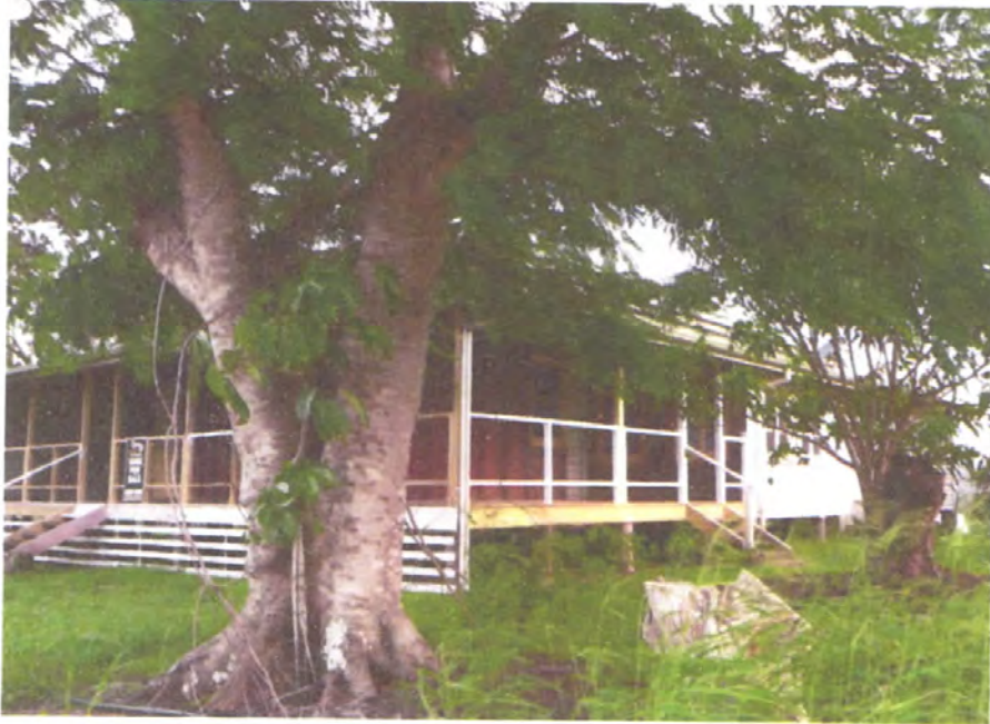
Figure 32 Mill managers house (September 2010)
