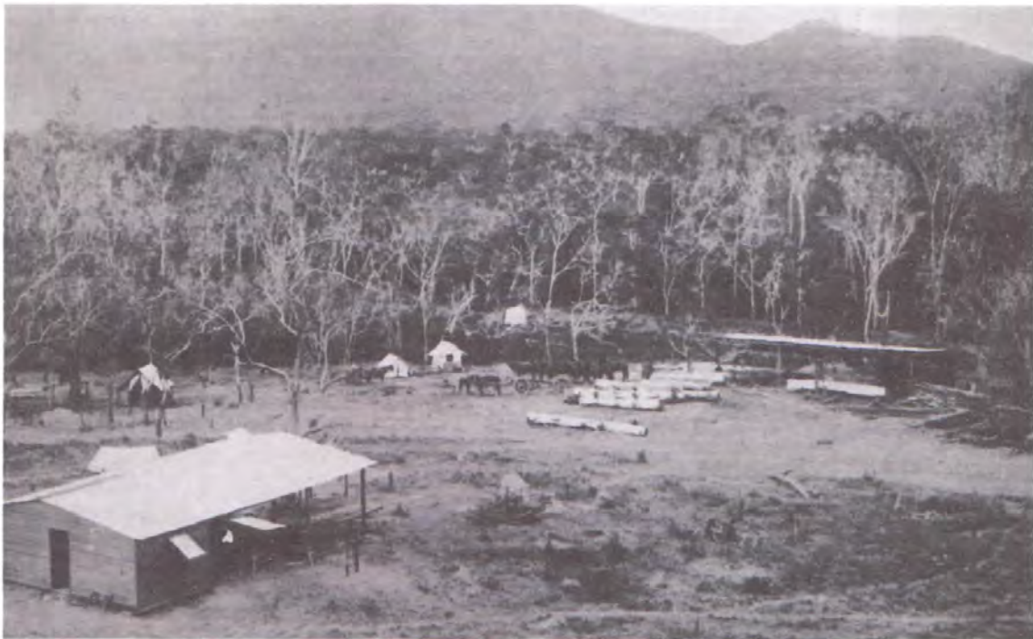
Figure 2 Sawmill at Mount Molloy Copper Mine, May 1905. The sawmill is to the right of the photo and shows a boiler and steam engine inside an open sided building. Logs waiting to be sawn are outside the building and to the right are off cuts and sawn timber (Queensland Government Mining Journal, 15 May 1905, p.220)
