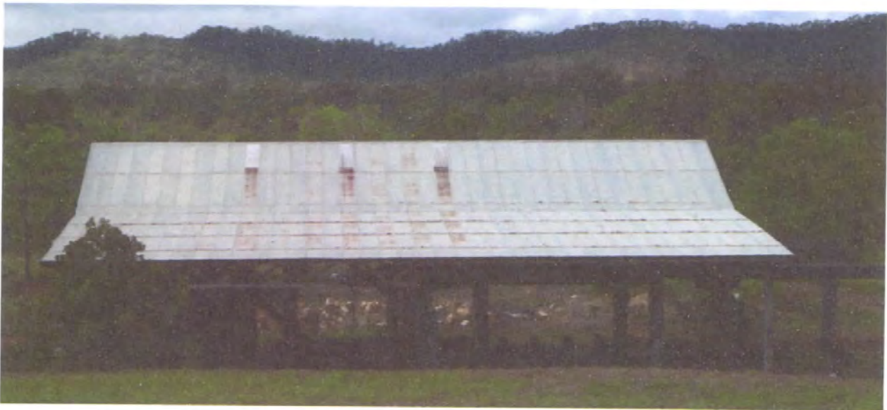
Figure 33 Electric sawmill building (September 2010)
