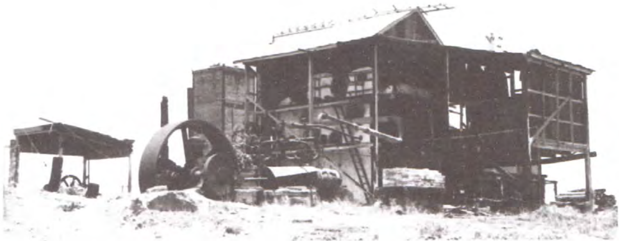
Figure 8 Mount Molloy sawmill in 1973, Marshall engine in the foreground, Walkers winch to the left in the background, and the boiler which was still protected by a building (Geoff Green, 1973)
